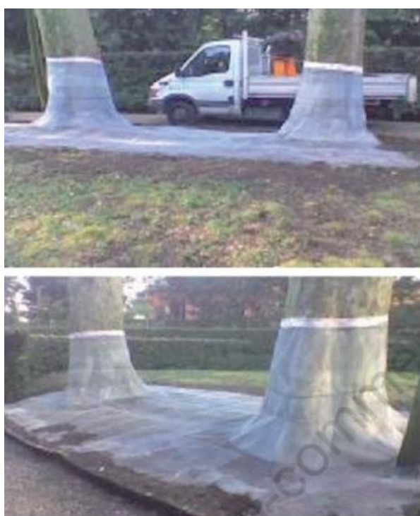
Figure 8-9. Wire mesh covering trunks and soil (using mosquito polyethylene net)
